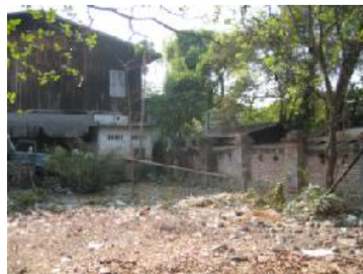
YMCA Nursery Mandalay: Construction Site
