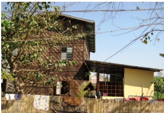
Annex (toilets, washroom, kitchen)
