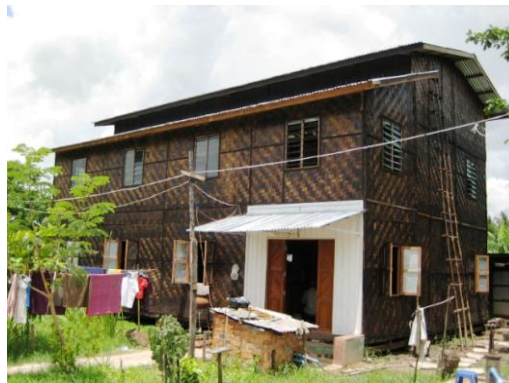
and after fitting walls and windows
