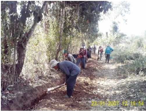
Water Pipeline Construction
