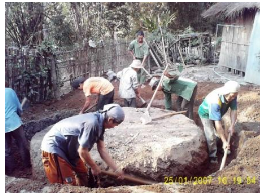
Water Tank Construction
