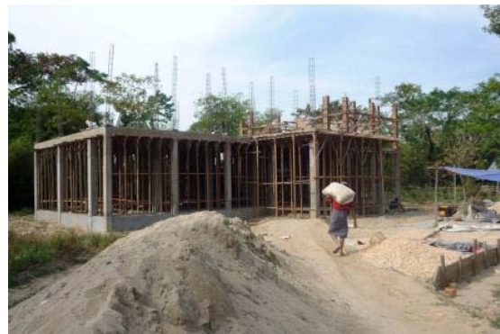
Magyikone Kyaiklat, Pathein (under construction)
