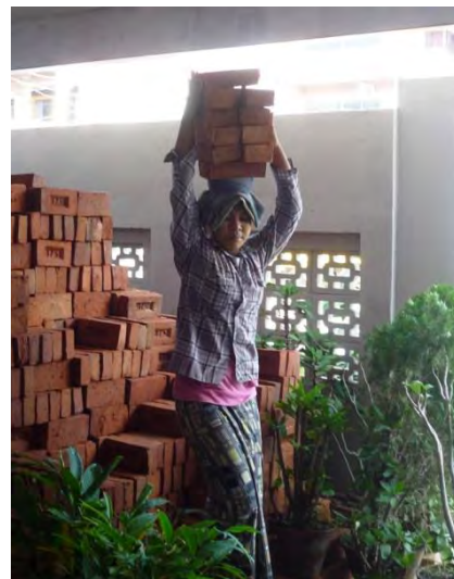
Heavy construction work is a women's job
