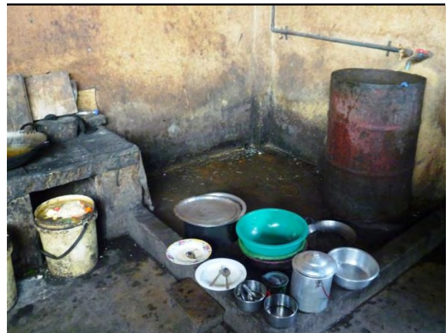
... and kitchen need urgent renovation
