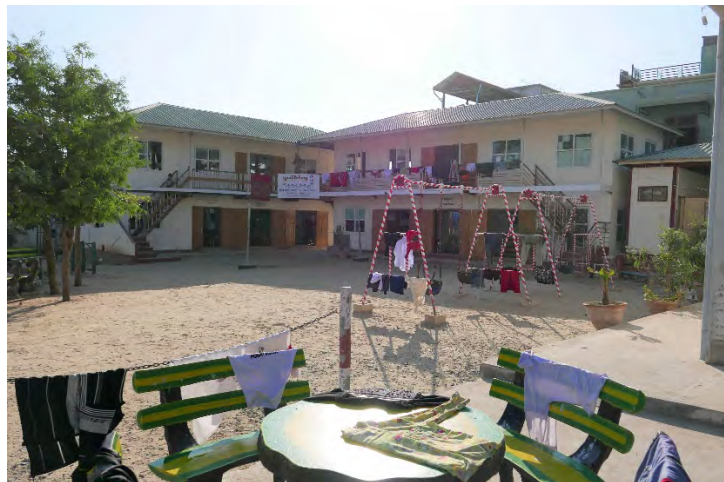
Temporary Shelter for Street Children
